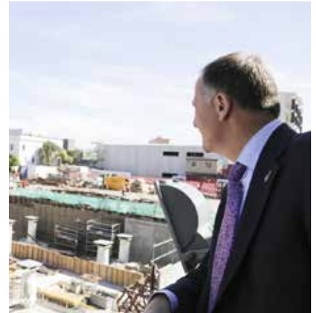
Prime Minister John Key observing the construction on Durham Street South
